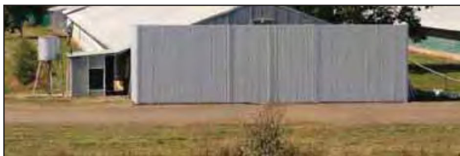
Figure 2.5 Windbreak wall constructed at a broiler shed.
