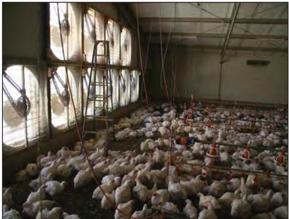
Figure 3.3 Interior of tunnel ventilated broiler shed equipped with large ventilation fans.
