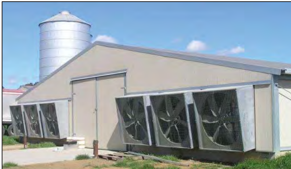
Figure 2.3 Tunnel ventilated shed used for poultry production showing extraction fans.
