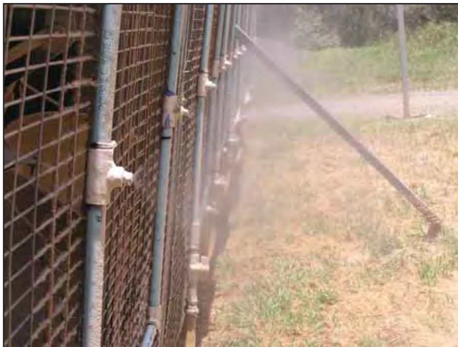
Figure 2.6 Application of liquid spray at the exterior of a ventilation fan.
