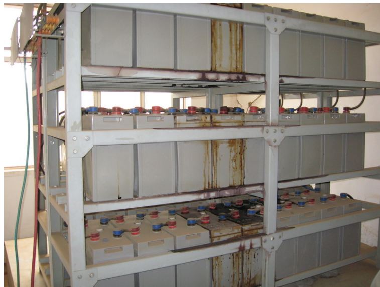
Figure 8.4: Township Electrification Program Battery Bank
