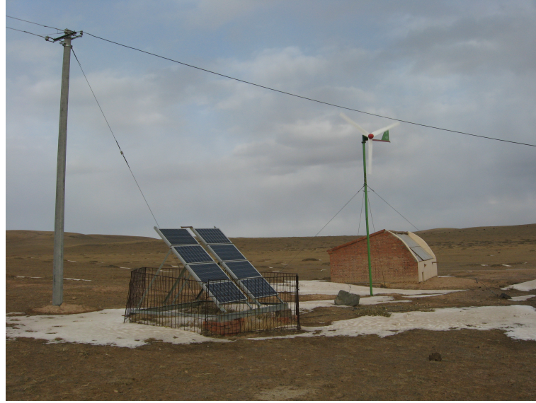
Figure 6.1: Brightness Program Wind and PV Components
