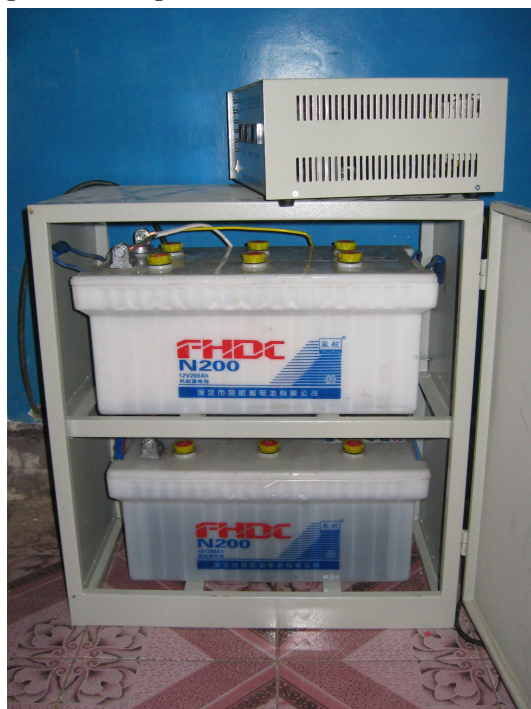
Figure 6.2: Brightness Program Pilot Inverter and Battery Components
