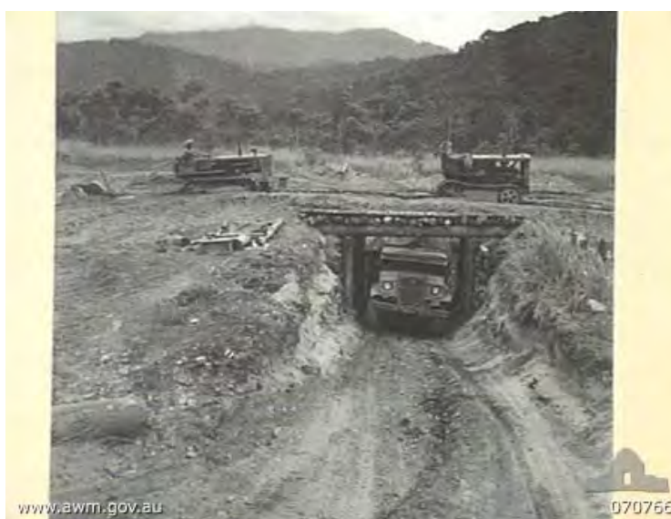
23. 1 March 1943 Chinaman loader at Wampit. This device is used to facilitate the loading of tip trucks.
