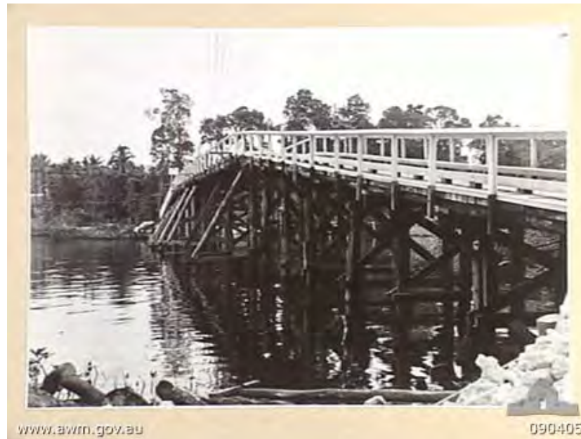
25. New Britain, 8 April 1945. Pile bridge over the Kalumalagi River built from local timber.
