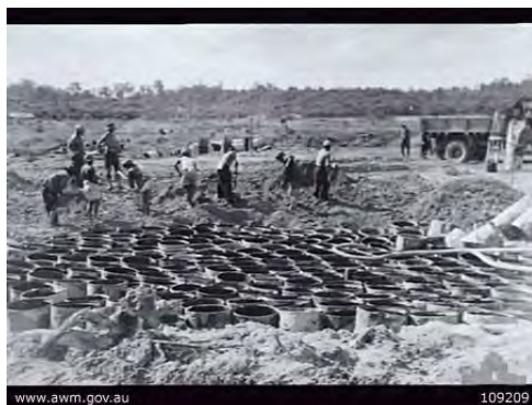
29. Tarakan, 4 June 1945. Civilians and No. 8 Airfield Construction Squadron fill a crater with gravel-filled drums
