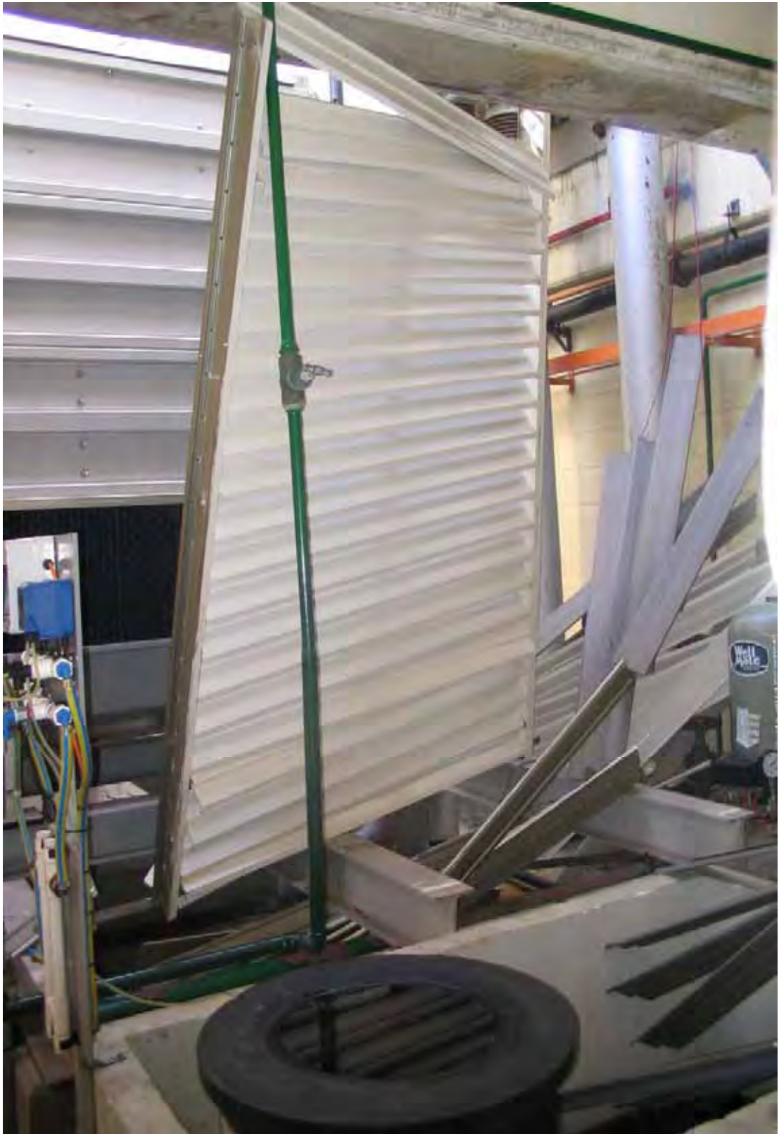
Figure 4.4 Louvre panels that have detached from structure above and fallen from level 29 down to level 28 in open section.
