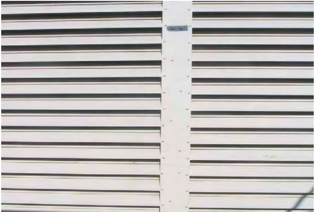
Figure 4.36 6061 T6 aluminium strip used to secure each louvre on site so as to obviate use of existing corroded screws; 6061 alloy strips placed only in centre of louvre system.
