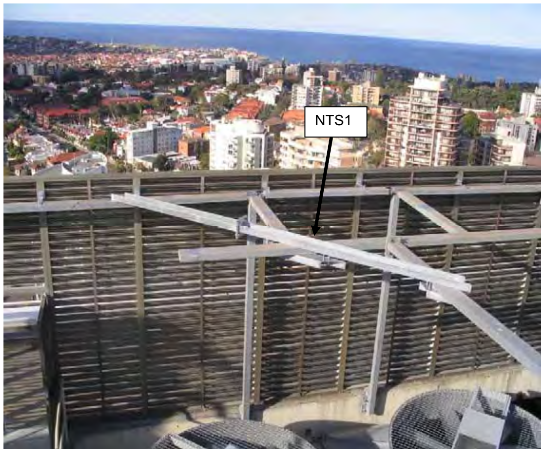
Figure 4.48b Top view of connection detail of cross beams (NTS1) and brackets using PFCs for additional strength on eastern face.
