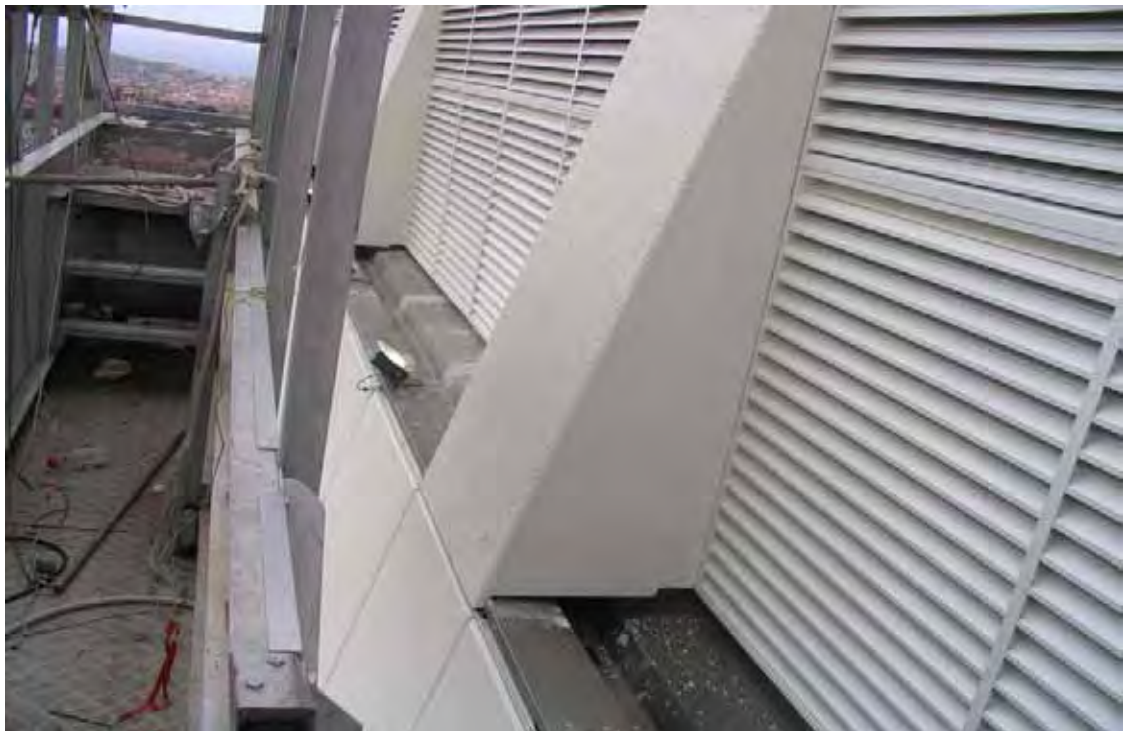
Figure 4.12 Difficulty in working on louvres at lower section, where steel cradle structure on left hand side is BMU.
