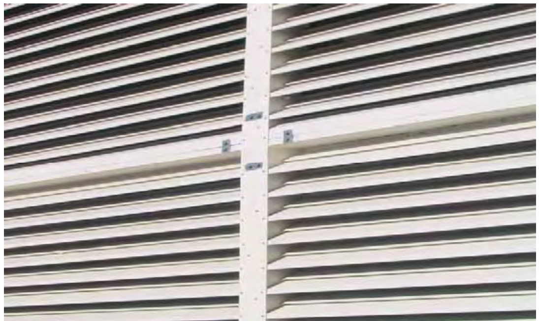
Figure 4.34 Louvre panels connected to internal bracket with high tensile M8 bolts.
