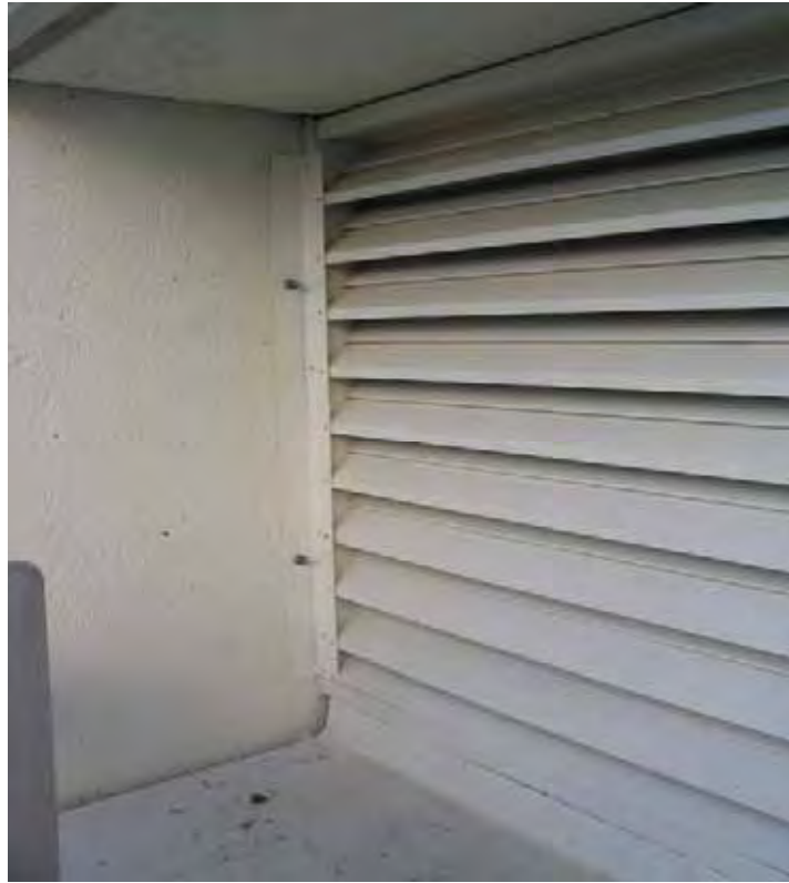
Figure 4.66e Aluminium equal angle 60 mm x 60 mm x 3 mm 6060 T5 chemically anchored to concrete wall and secured to louvre as in levels 27 and 28.
