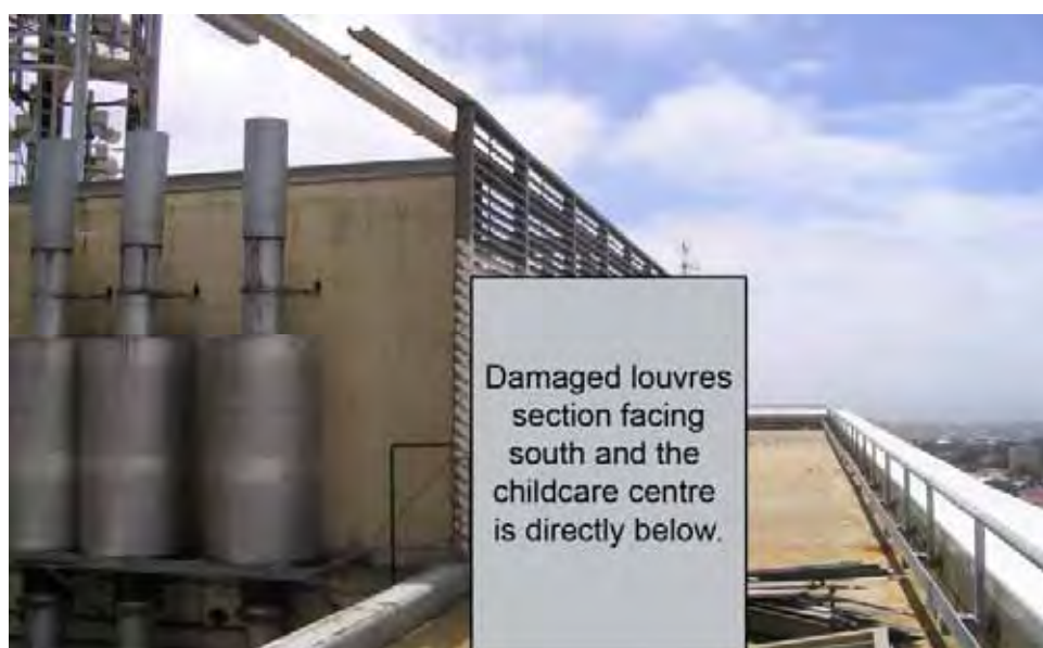
Figure 4.14 Damaged louvre section on southwest corner of roof on level 29.
