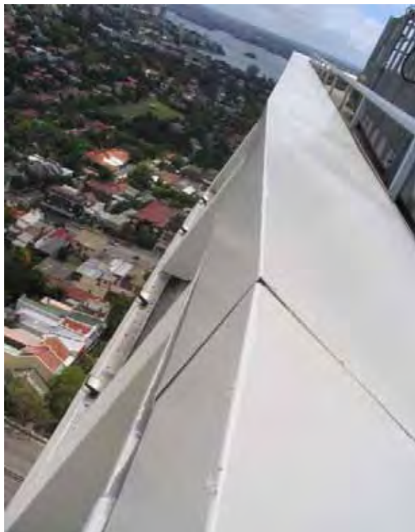
Figure 4.56 Typical cladding separation from mullion sections throughout.
