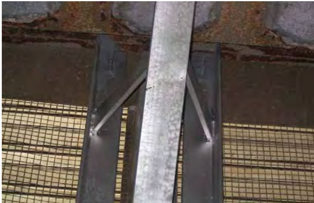
Figure 4.65b Upper U-bracket connecting mullion in internal of level 28 using bolts specifically threaded to account for extra length, enabling abseilers to use specially made jigs to drill through mullions and bolt directly through welded nut on brackets.
