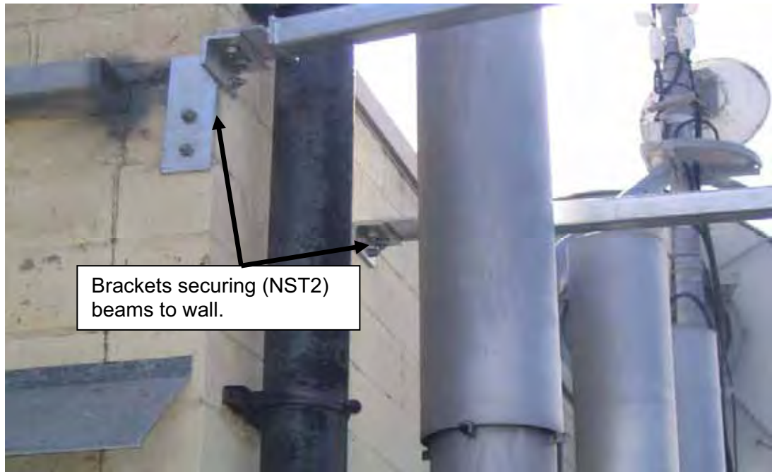
Figure 4.47 Intricate connection of brackets to wall using chemical anchoring.
