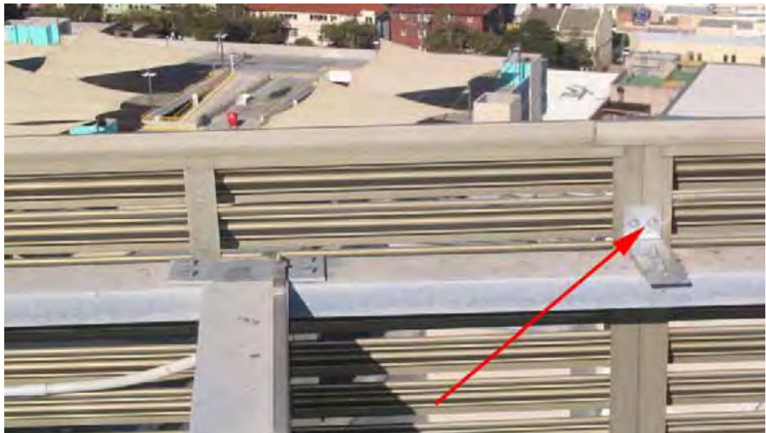
Figure 4.31 Typical connection for each bolt in each vertical mullion.
