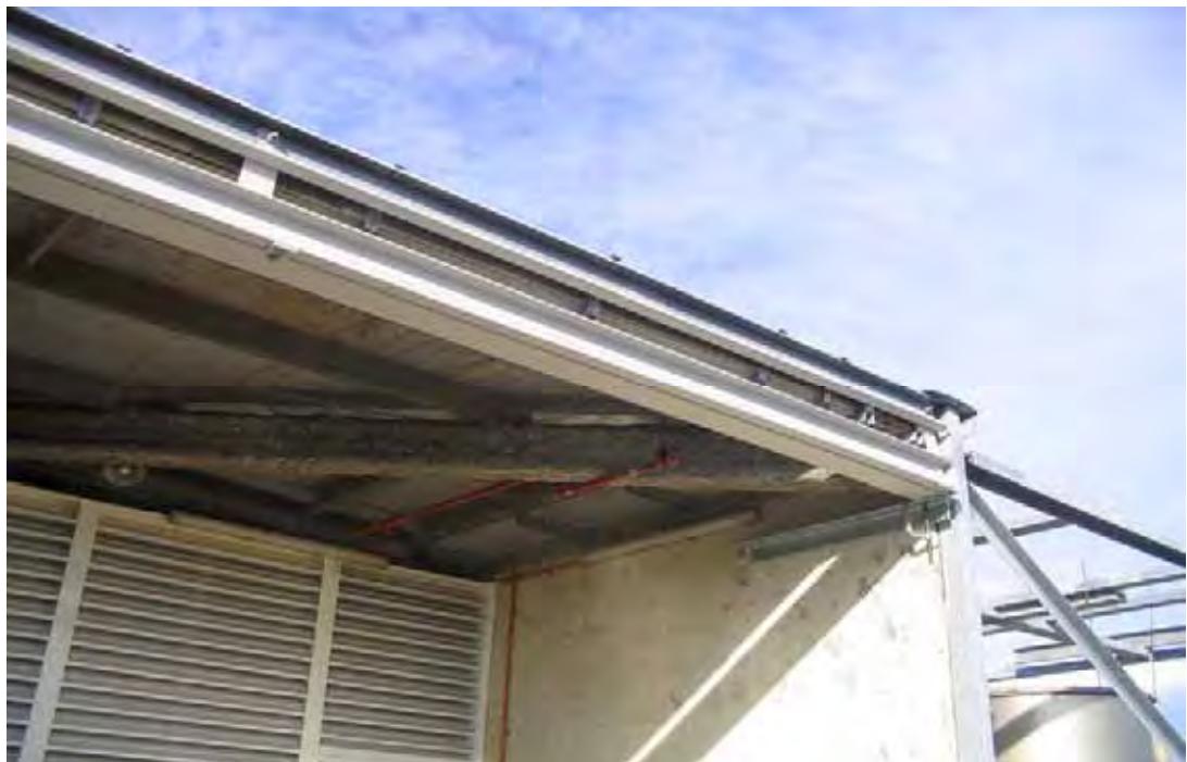
Figure 4.25b Refurbished beam with Emerbond and Emerclad and new hot dipped galvanised support from below.
