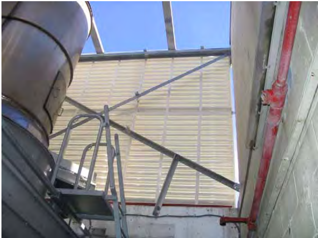
Figure 4.51 Several additional hot dip galvanised brackets and connections utilised to give further strength to western side.
