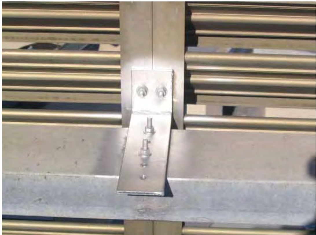
Figure 4.29b New hot dip galvanised brackets designed for optimal strength, connected with structural galvanised M8 bolts through mullion and into bracket; structural galvanised M8 bolts connecting bracket to PFC.
