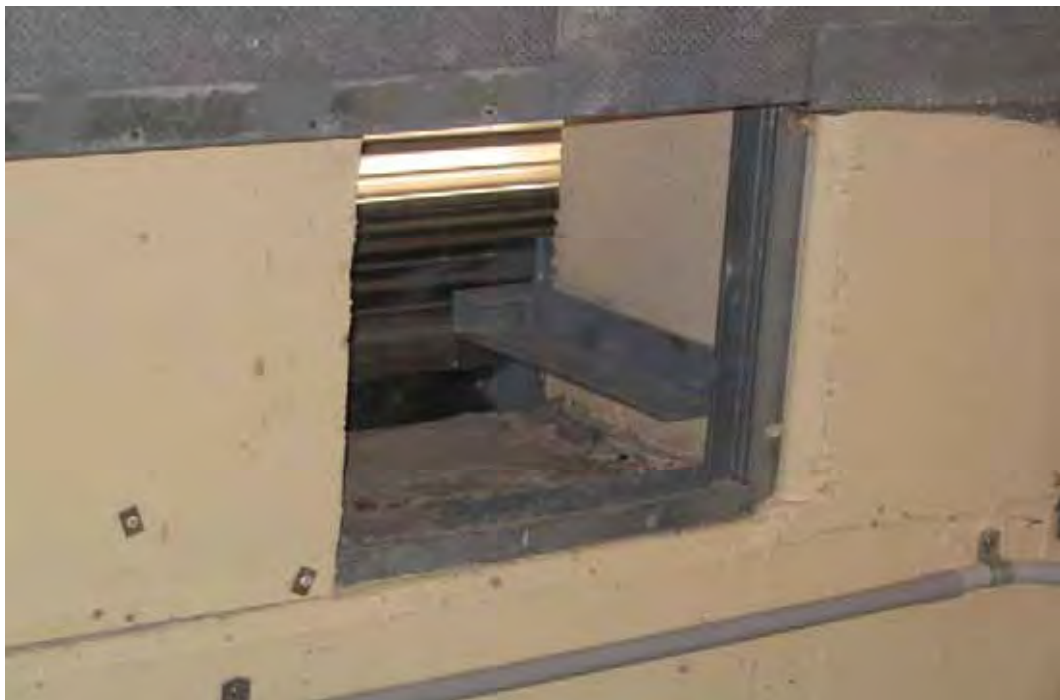
Figure 4.65d Detail of plate (for lower bracket) sitting behind hob and awkward to access.
