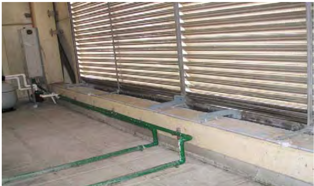
Figure 4.22 Brackets placed in four locations to provide extra support and replace older brackets.
