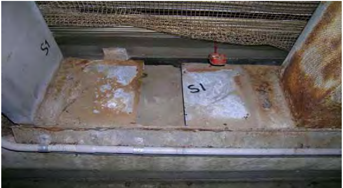
Figure 5.5 South section; fully under cover; with plant in front; corrosion commencing; westerly wind impinging on plant in front of section and on semi-wall in front of section, protecting it from excess airborne contaminants.
