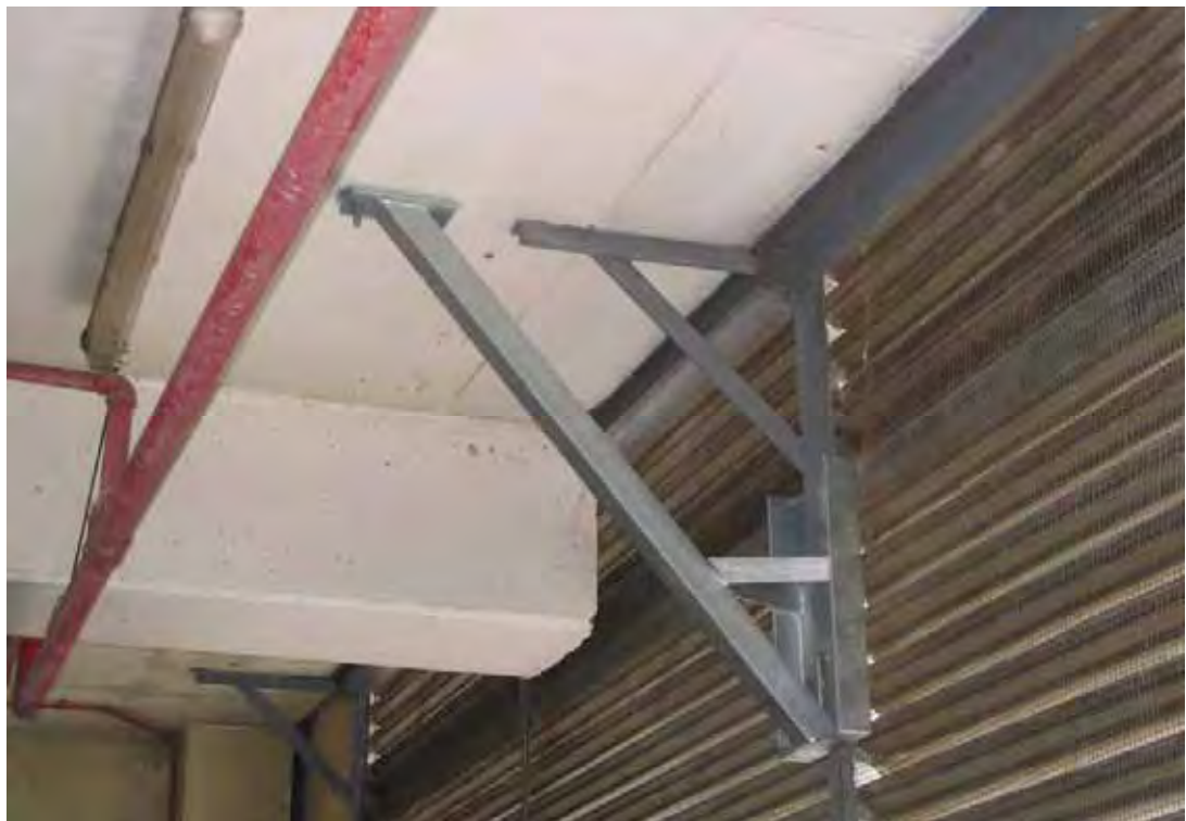
Figure 4.20 Typical U-shaped brackets fabricated and hot dip galvanised for upper sections of louvres on level 28.
