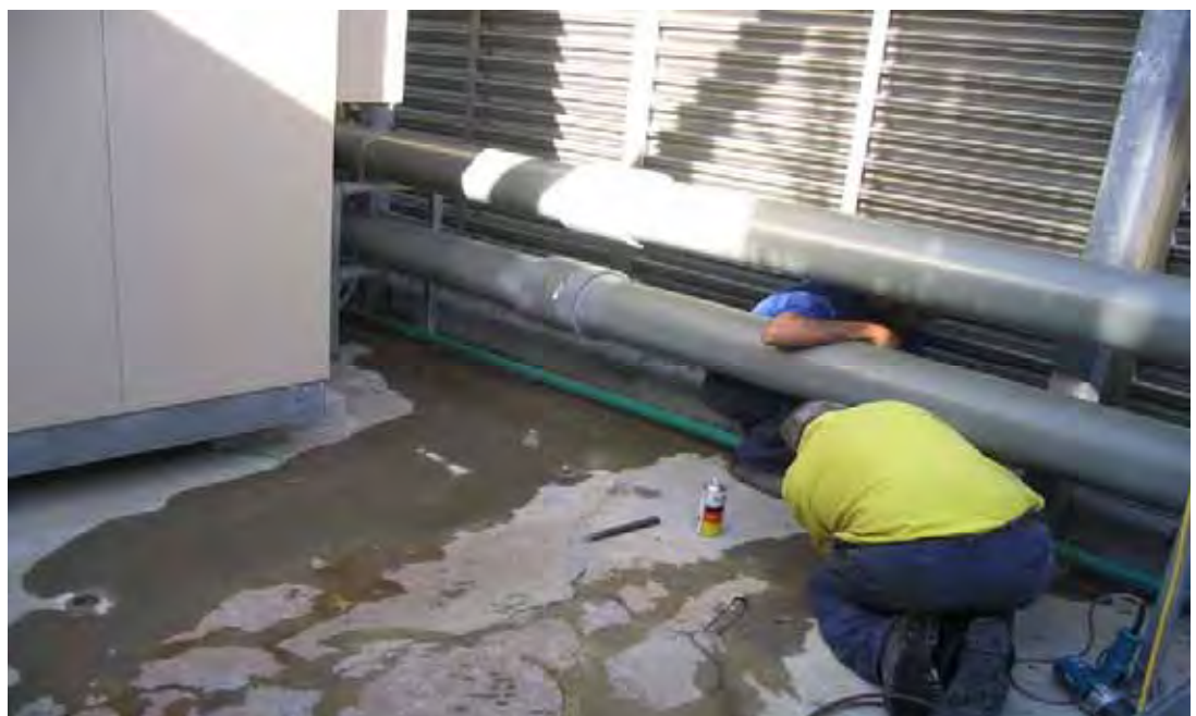
Figure 4.42 Water draining from columns due to drilling at base of each of columns to allow bleeding of excess water.
