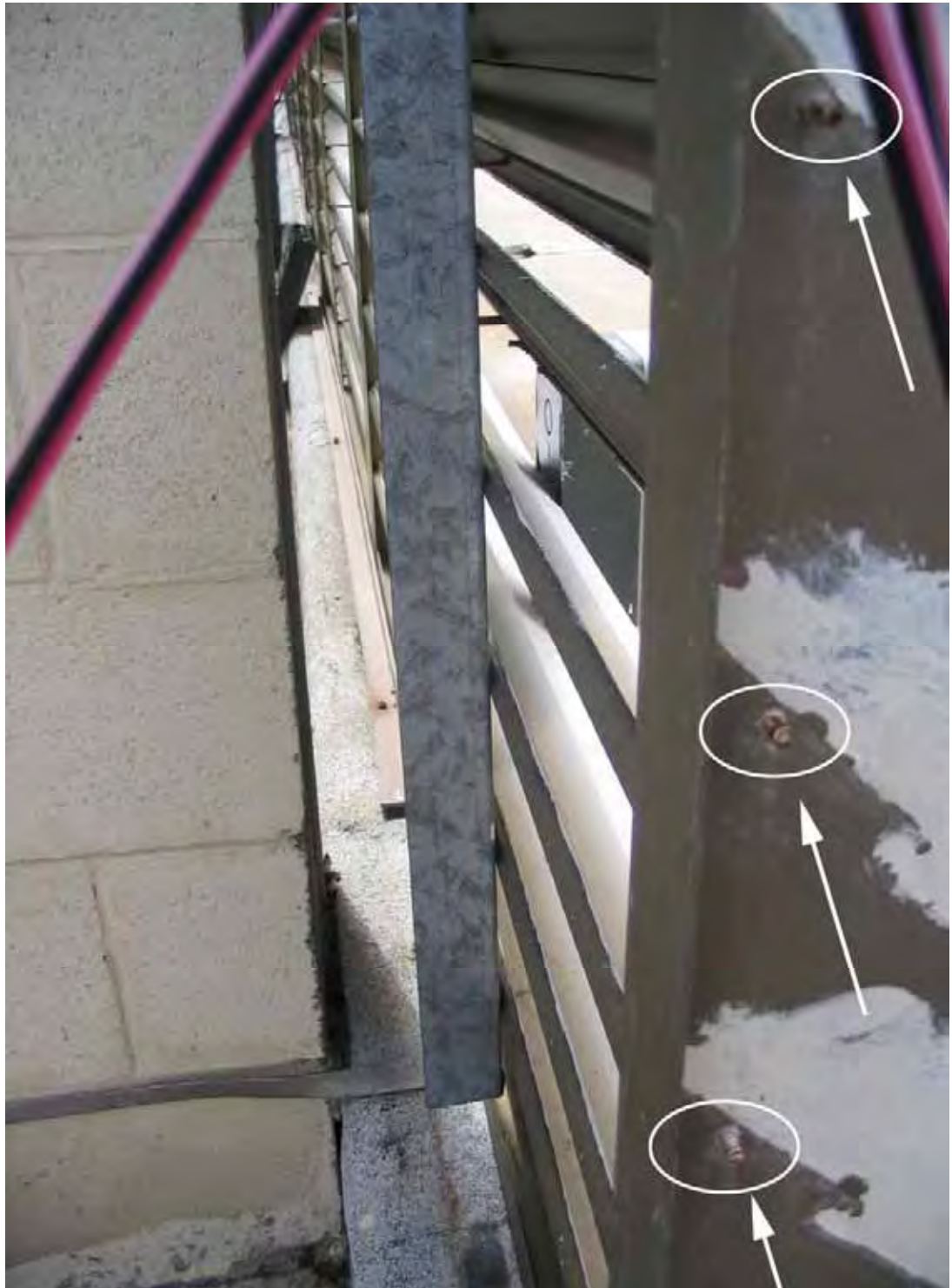
Figure 4.35 Corroded screws typical of all existing Westfield louvre connections in mullions.
