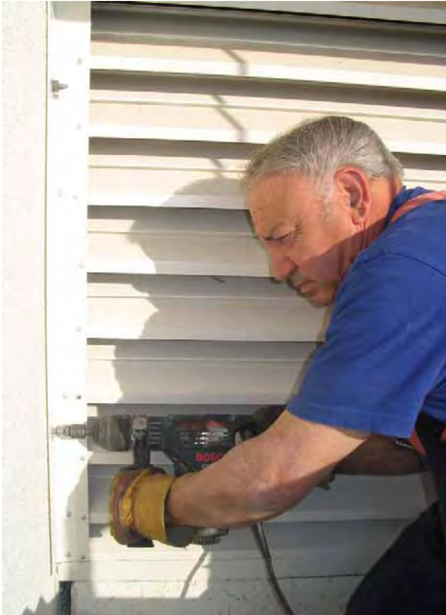
Figure 4.68 Typical concrete drilling to secure aluminium equal angles and chemically anchored to concrete on both walls and roof of level 26 anchored to concrete roof to hold louvre mullion sections in centre.
