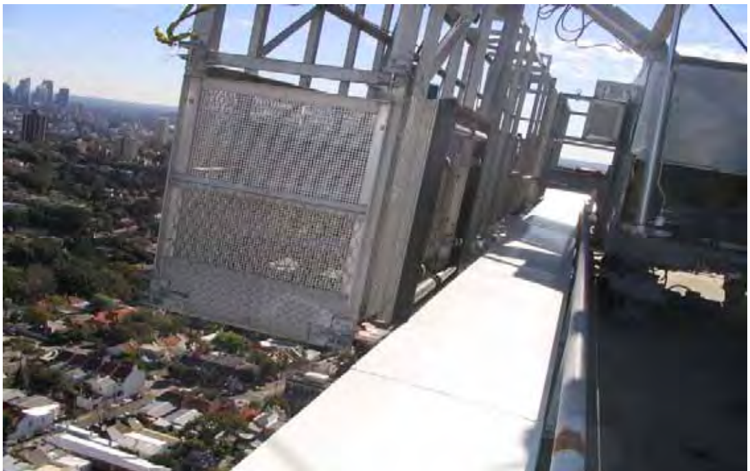
Figure 4.59 Potential of BMU to descend posing serious structural problem for integrity and life of cladding.
