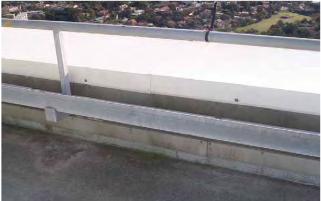
Figure 4.55 Typical section of cladding on level 29, showing M8 dynabolts fixed to concrete hob using washers to avoid tearing effect; galvanised bolts placed all around parapet with appropriately sized galvanised washers.
