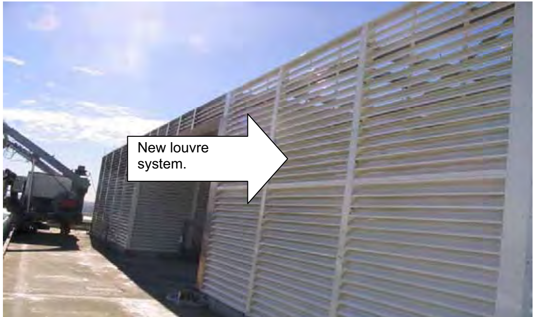
Figure 4.49a New southwest louvre section; each louvre fully welded to mullion and powder-coated.
