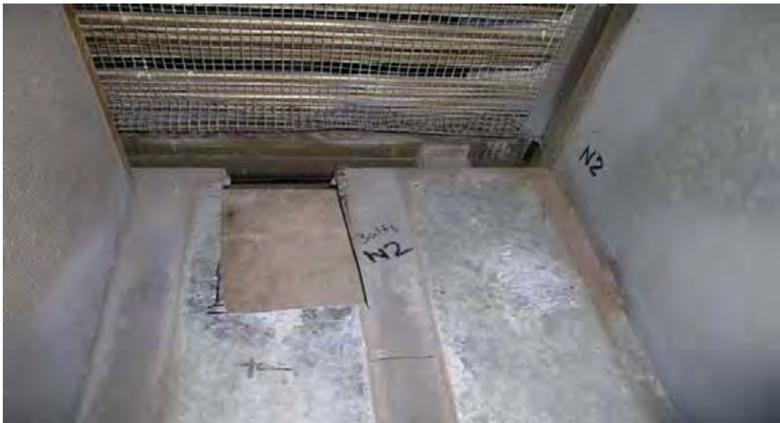
Figure 5.4 North (N2); level 28, showing condition of both baffles on sides and louvre in centre in nearly acceptable state; fully covered; all sides fully enclosed by concrete walls; only open position from louvres facing outside; resulting in no corrosion.
