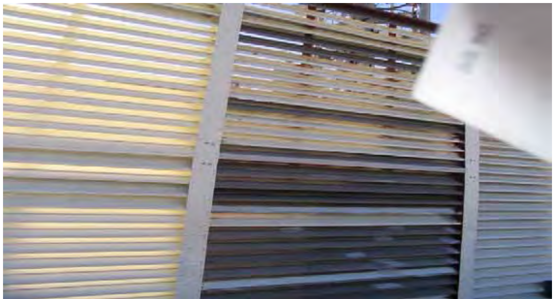
Figure 4.50b Panel section facing south as fabricated using existing louvres.
