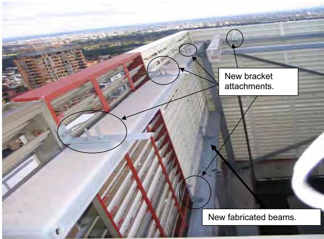
Figure 4.50a Panel section (with red primer) facing south fabricated fully using existing louvres.
