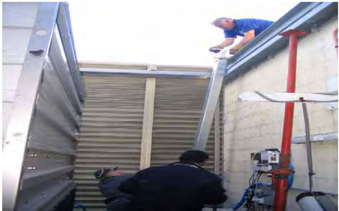
Figure 4.40 New hot dip galvanised RHS replacing old corroded column shown in figure 4.39; holes on top for galvanising were sealed with two-mix steel putty.
