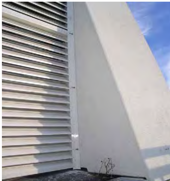
Figure 4.66d Aluminium equal angle 60 mm x 60 mm x 3 mm 6060 T5 (bottom section) chemically anchored to concrete wall and secured to louvre panels using riveting.
