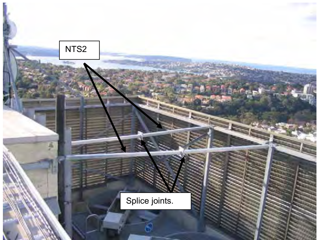
Figure 4.46 Hot dip galvanised cross beams (NTS2) and brackets designed to provide further structural support for eastern section of louvres.
