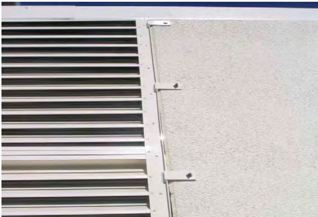
Figure 4.66b Aluminium unequal angle 60 mm x 25 mm x 3 mm 6060 T5 (top section) riveted to louvres and welded to unequal angle 100 mm x 50 mm x 6mm 6060 T5 brackets, which were chemically anchored in concrete wall.
