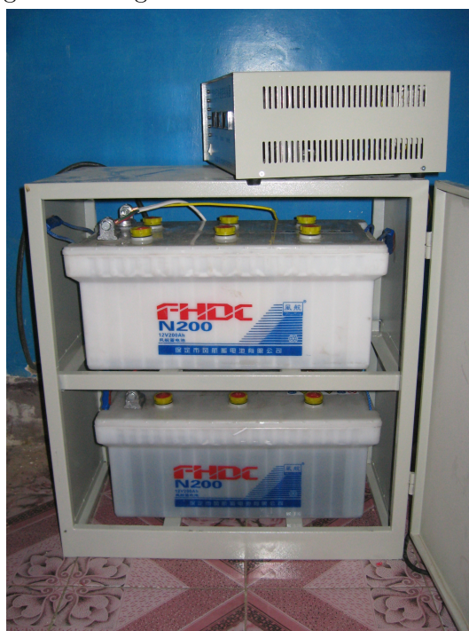
Figure 6.2: Brightness Program Pilot Inverter and Battery Components
