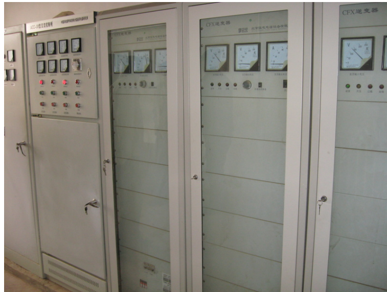
Figure 8.3: Township Electrification Program Inverters and Charge Controllers
