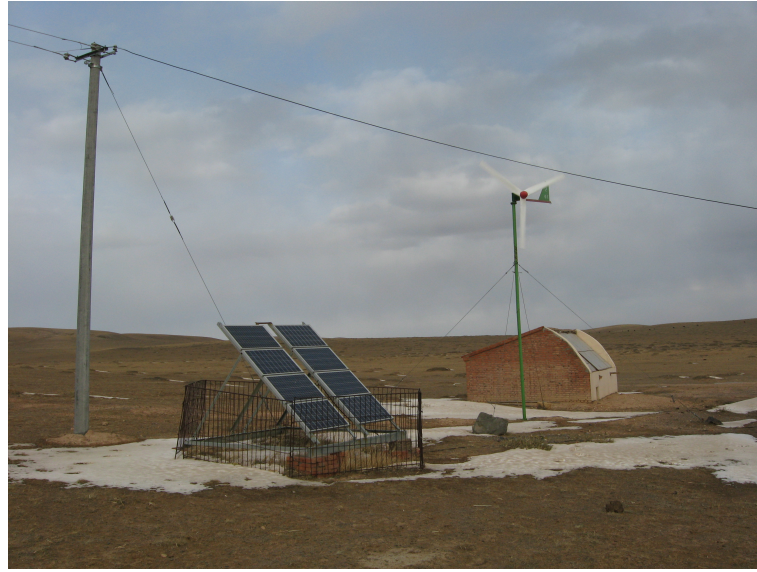
Figure 6.1: Brightness Program Wind and PV Components
