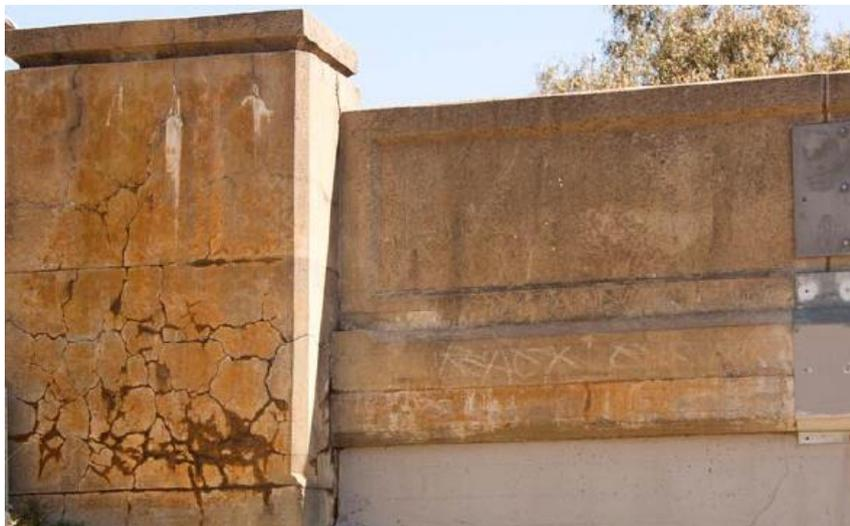
Figure 2-9 : Map cracking due to alkali silica reaction identified in causeway bridge in Perth (Australia 2015)
