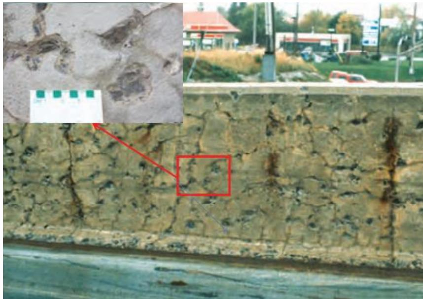
Figure 2-10 : Surface pop outs due to alkali aggregate reaction (Thomas et al. 2011)
