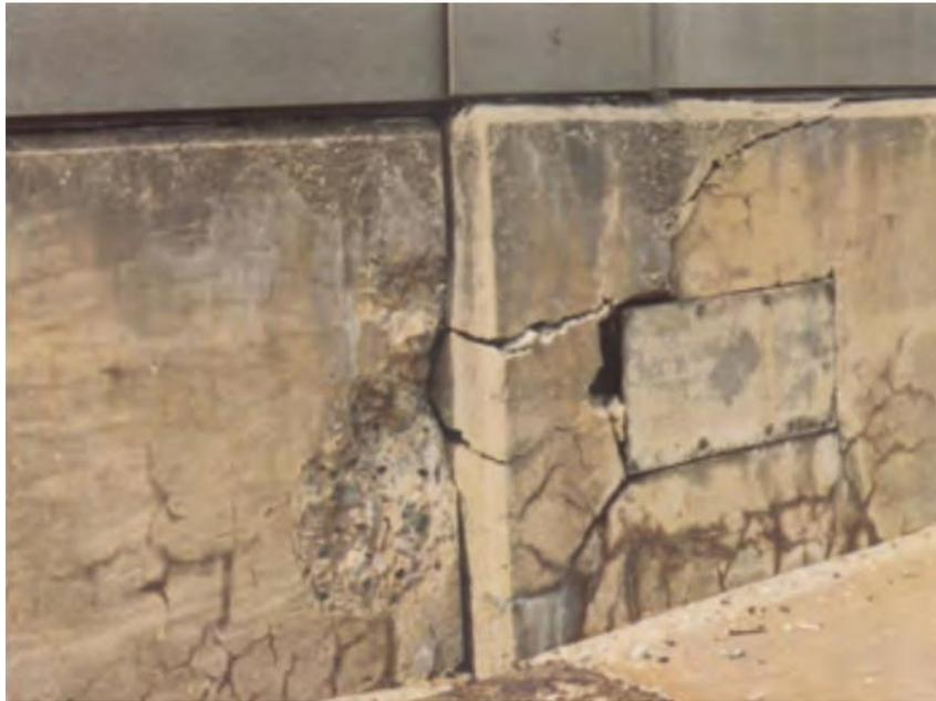
Figure 2-11 : Differential movement of parapet walls in a bridge due to AAR (Thomas et al. 2011)
